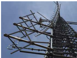
Our 3-bay circular polarised antenna at Acacia Rd, Somersby
